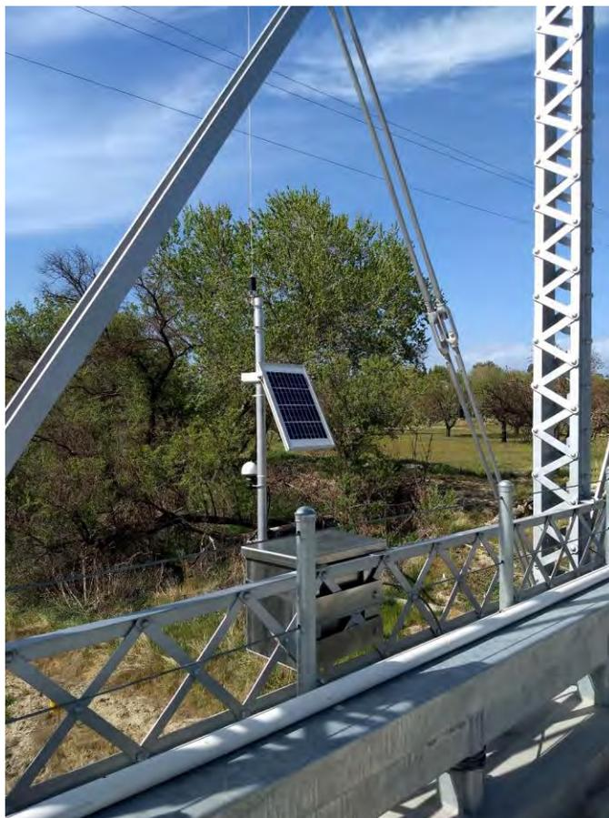
*Figure 2. Whitley Gardens (Estrella River) radar sensor stream gage installation*
