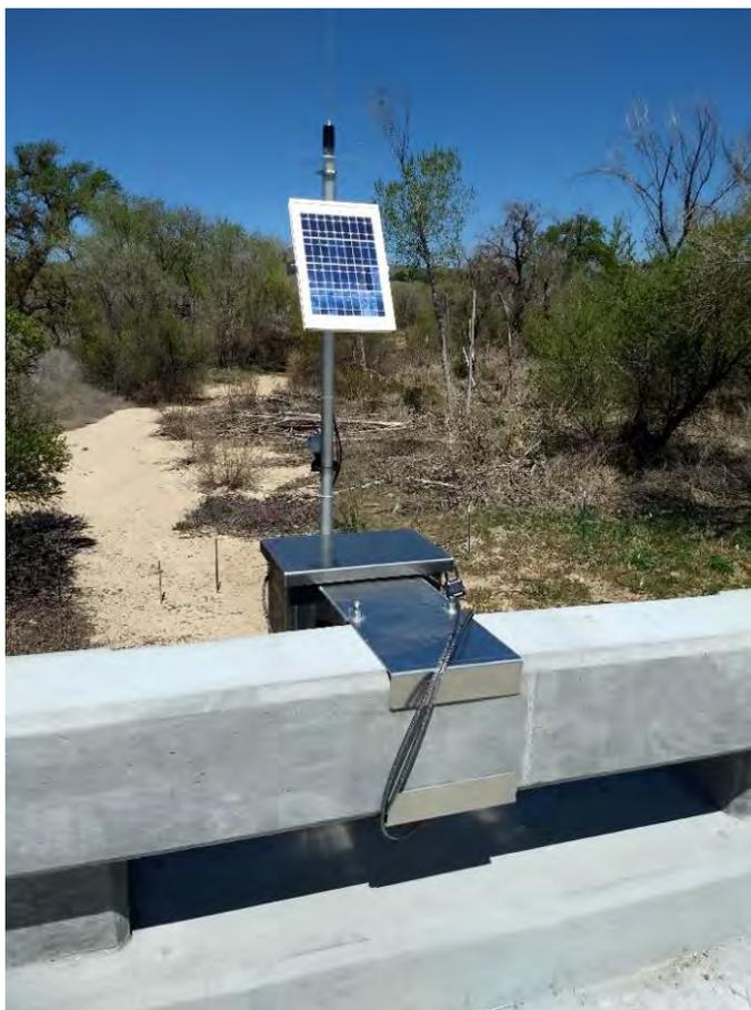
*Figure 4. Creston (Huer Huero Creek) radar sensor stream gage installation*
