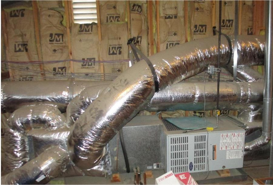
Figure 2.12: Carrier 6-ton Air Handler in Attic of District Office
