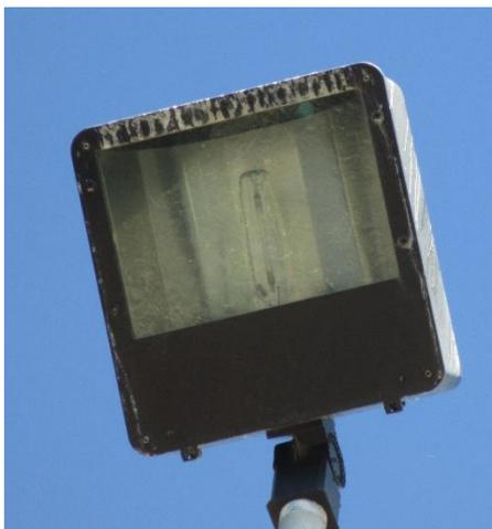
**Figure 2.10: Typical HPS Pole-Mounted Fixture at WWTP**
