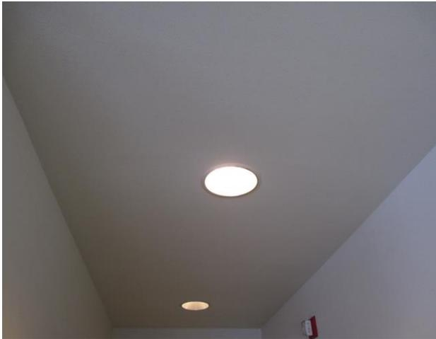
Figure 2.7: Hallway CFLs
