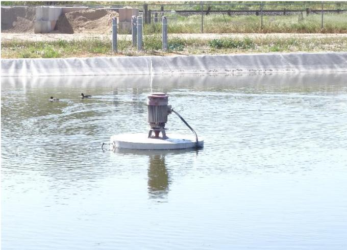
Figure 4.3. Surface Mechanical Turbine Aerator in Pond 1
