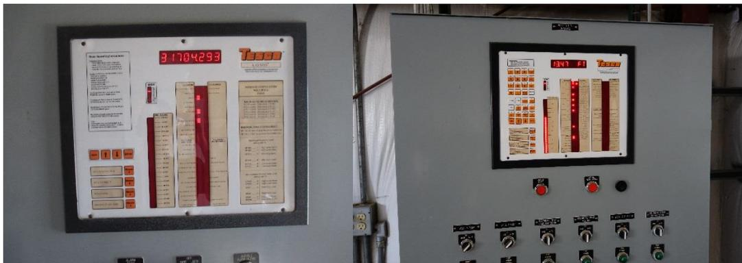
**Figure 4.5. Well #3 Pump Controller (left) and Well #4 Pump Controller (right)**
