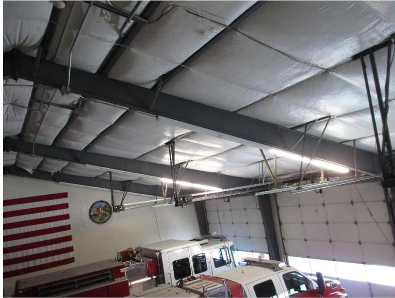
**Figure 2.9: New Firehouse Engine Bay Fluorescent Fixtures**
