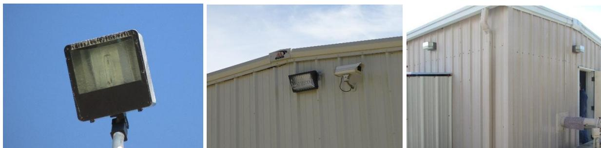
Figure 4.2. WWTP HPS (left), WWTP MH wall pack (center), Well pump 4 MH wall packs (right)
