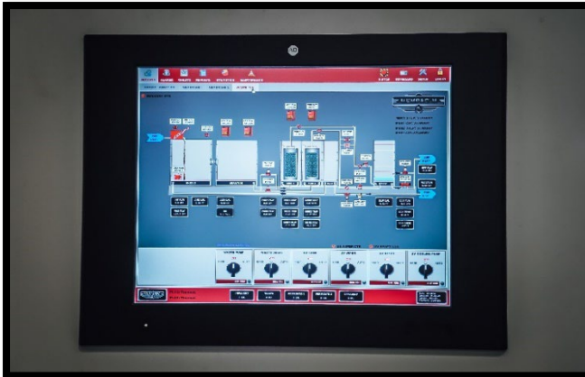
Figure. Clearwell and Membrane chamber and electrical control equipment (provides remote access).
