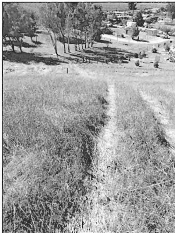
Photo 4. Water line route, view southwest. 11/3/2016.
